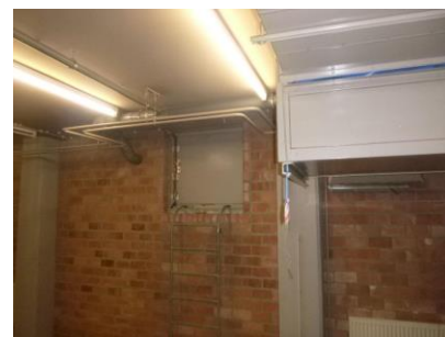
foto: brandwerende beplating
