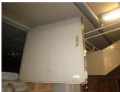
foto: brandwerende beplating
