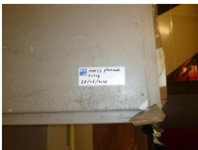
foto: brandwerende beplating
