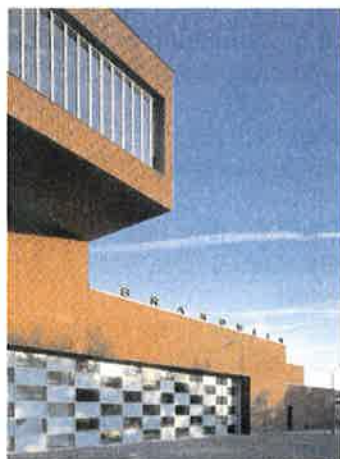
Brandweerkazerne, Breda Architect: Neutelings Riedijk
